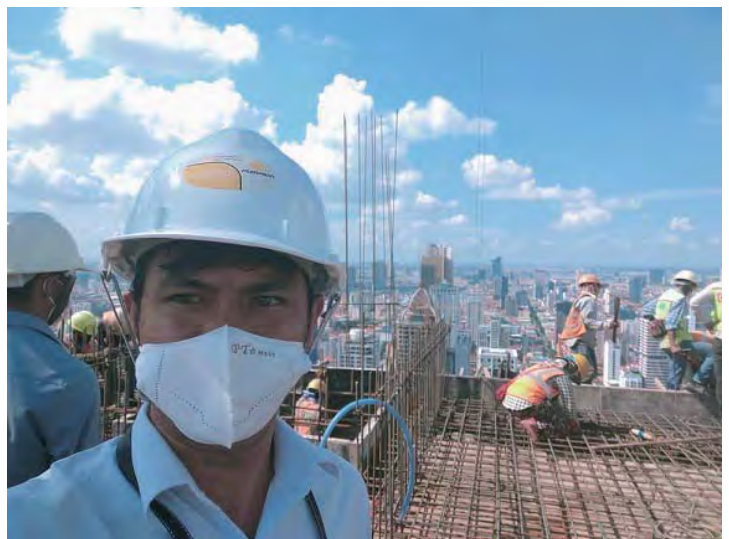
Mr. Chamnab Voeun (at the construction site of a condominium in central Phnom Penh).
